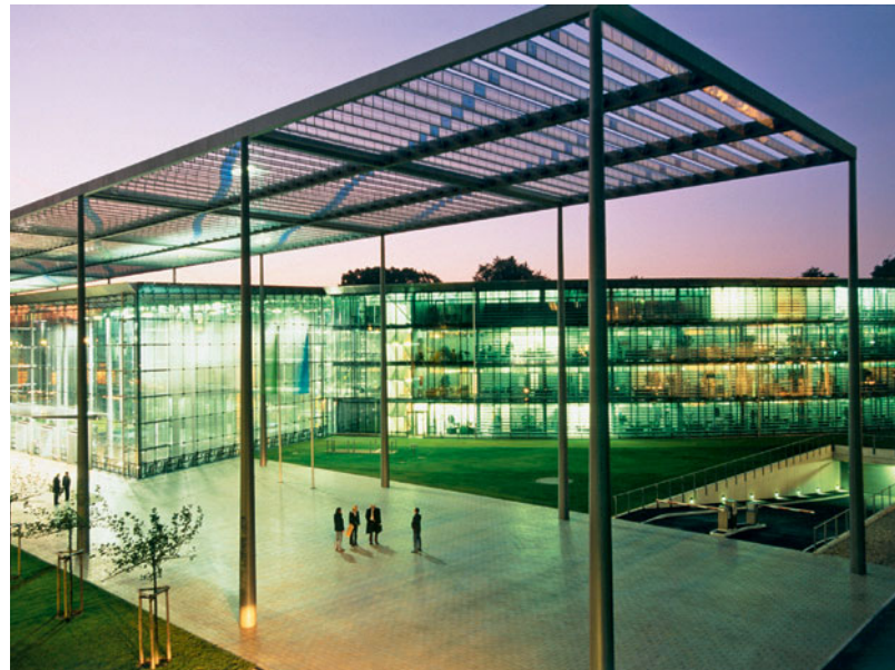
Bayer AG headquarters in Leverkusen
